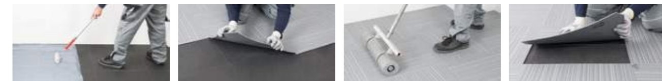
Installation with tackifier
